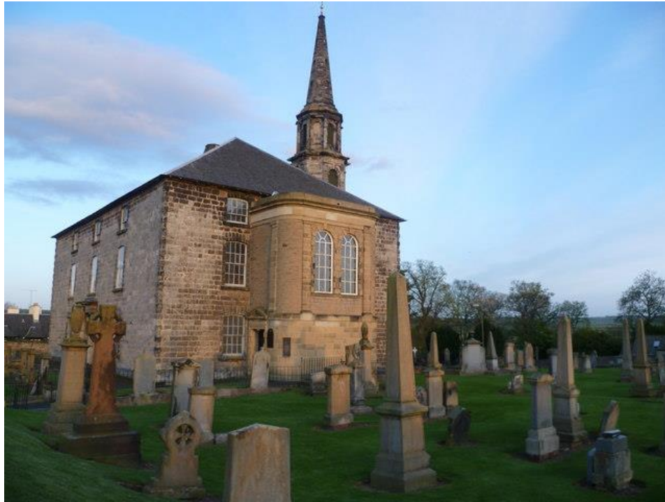
St. Michael's Parish Church, Inveresk, Scotland (Photo by Kim Traynor)
